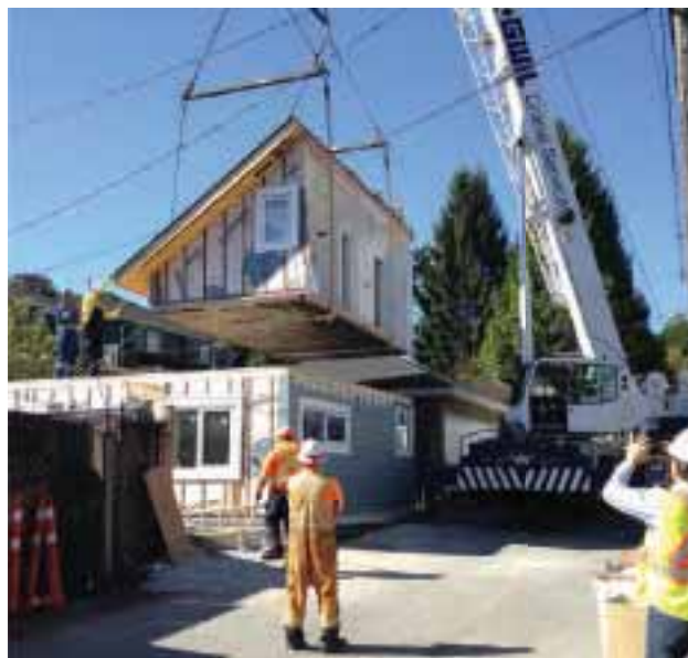
Modular units create a My Lane Home laneway house in Vancouver: faster and cheaper to build, with less disruption to the neighbourhood. | MY LANE HOMES
