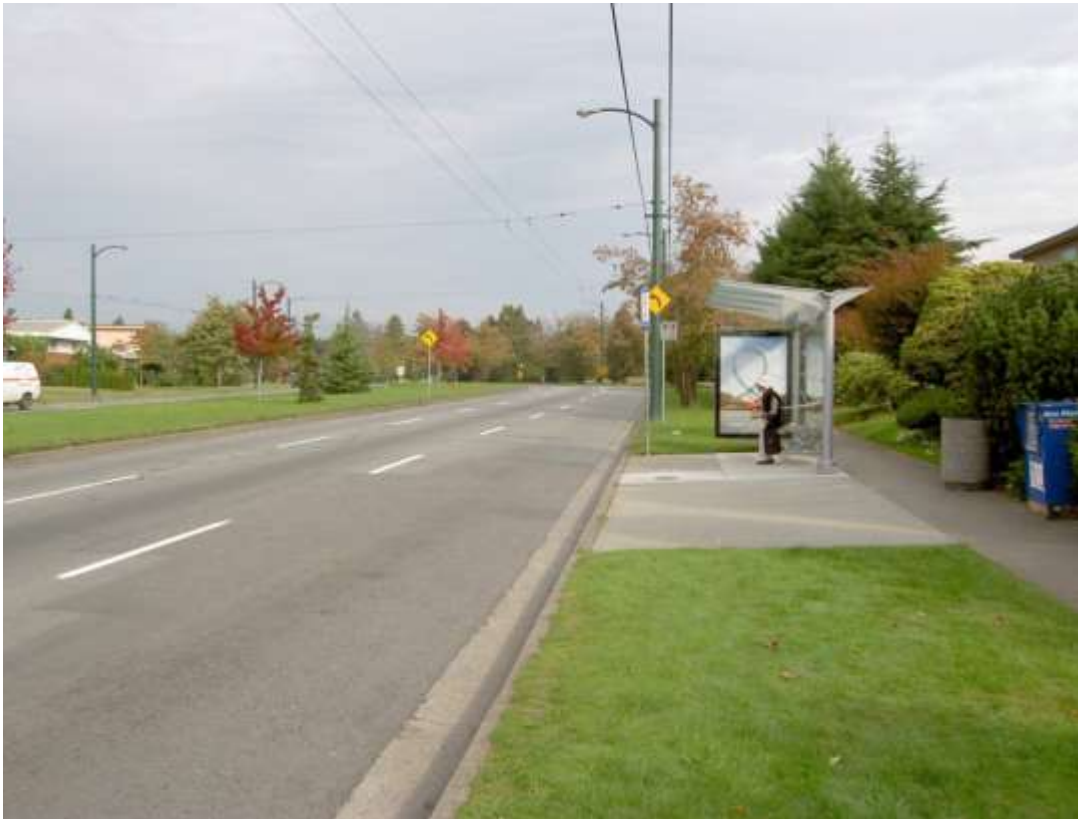
The bend to 37th Avenue, looking North
