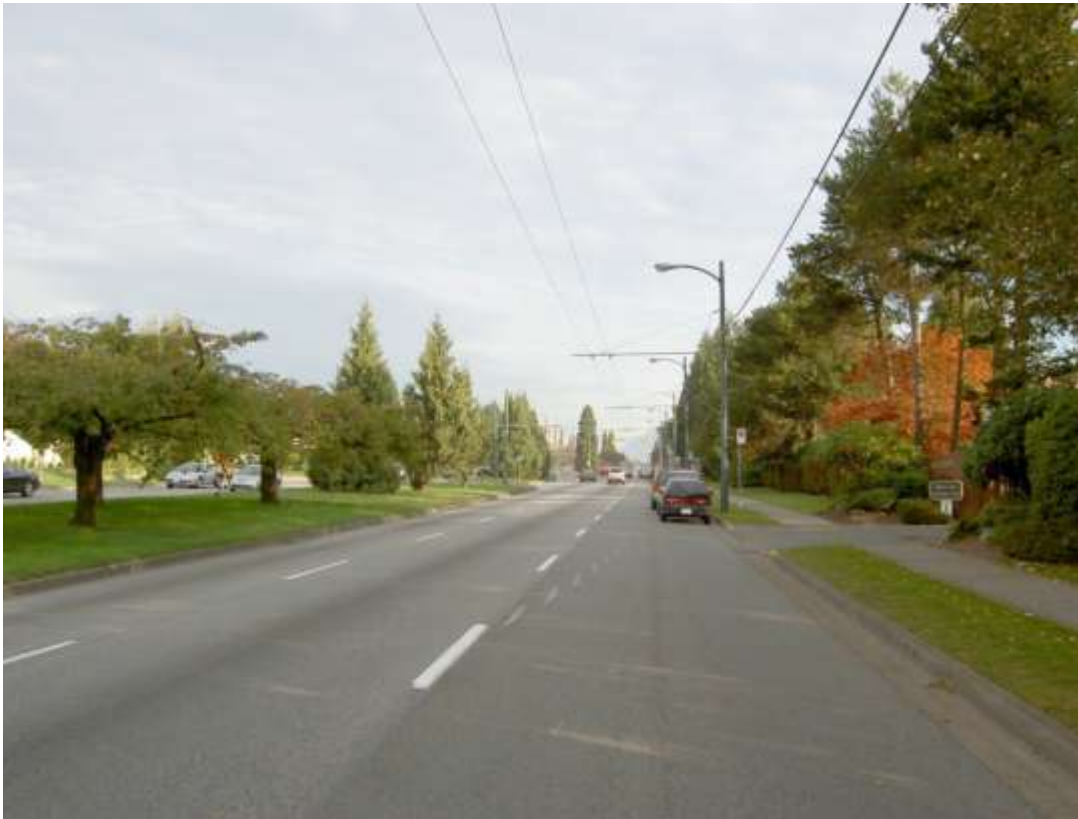
49th Avenue to 54th Avenue, looking North
